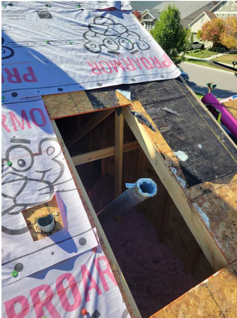
28 1-water soak decking replace Date Taken: 10/8/2024
