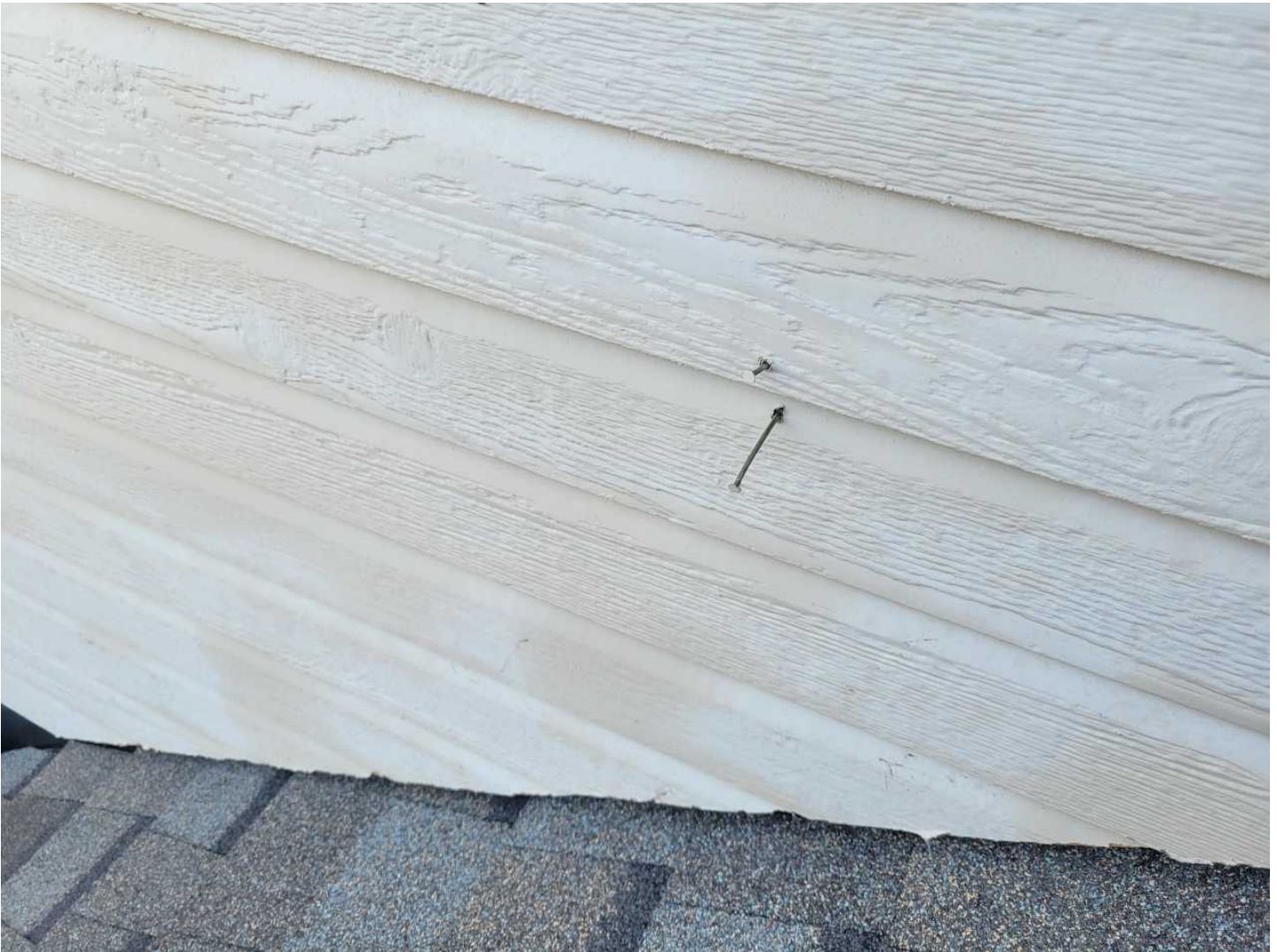
22 23-roofer hours to renail siding Date Taken: 10/25/2024
