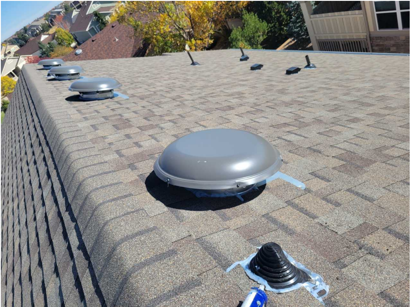
26 27-split boot to seal roof anchors Date Taken: 10/25/2024
