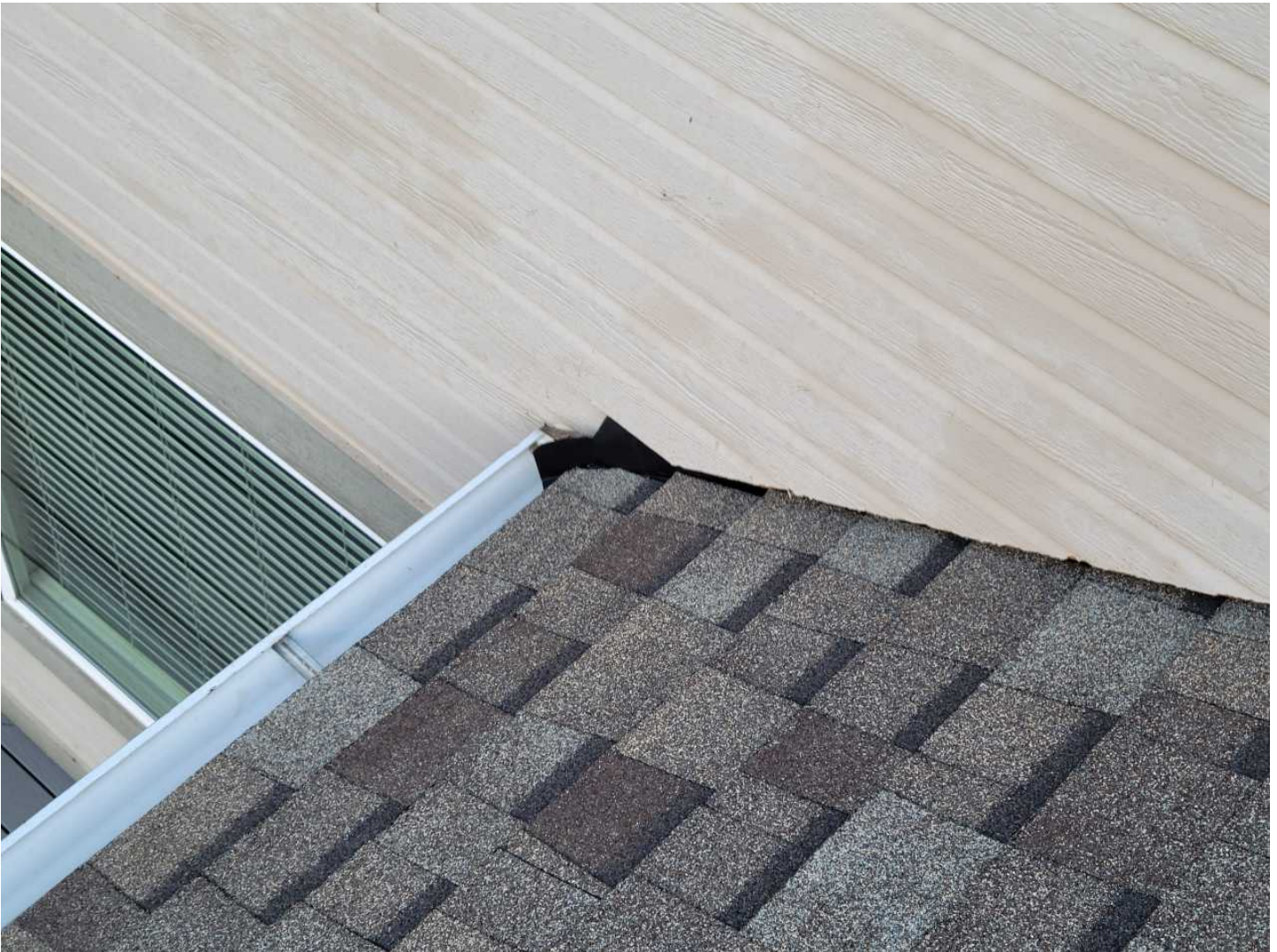
15 16-kickout flashings as existed Date Taken: 10/8/2024
