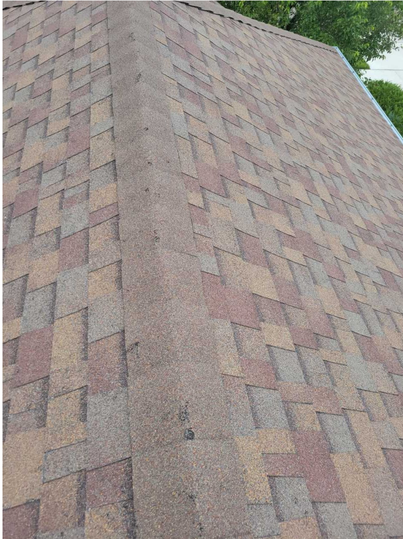
13 14-high profile ridge as existed Date Taken: 6/24/2024
