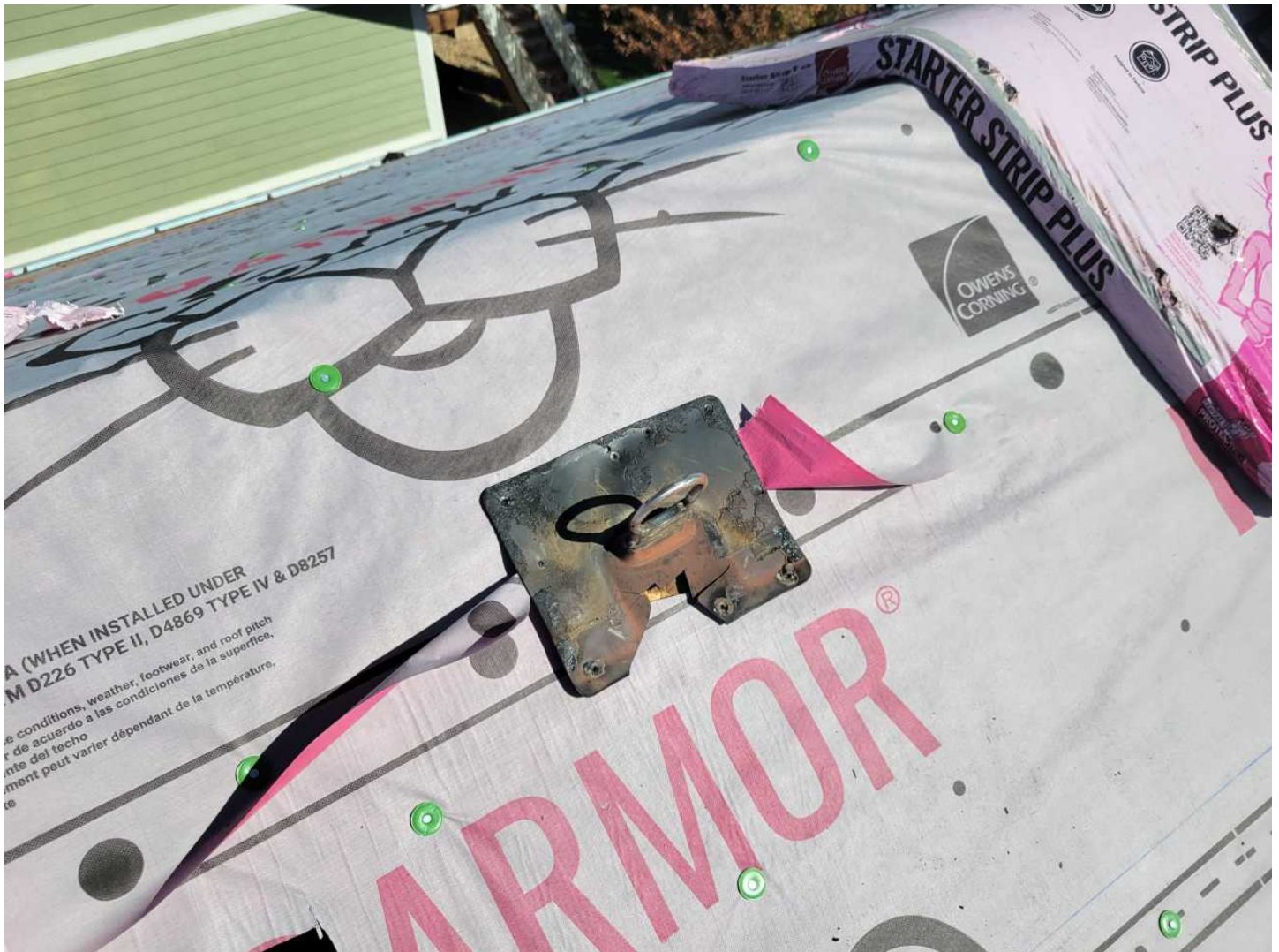
21 22-reuse reseal anchors
