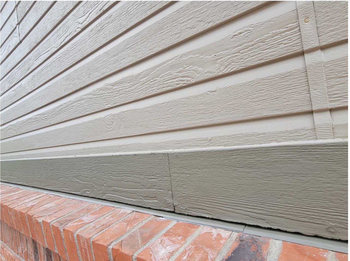
17 18-paint trim left elevation(1) Date Taken: 6/24/2024
