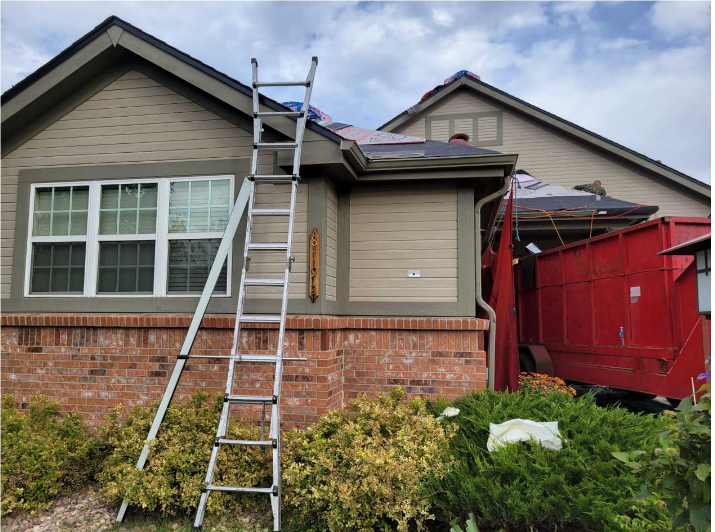
12 13-haul away with light weight rubber tire contr Date Taken: 10/8/2024
