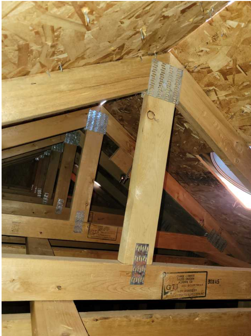
8 9-electrical disconnect vent remove Date Taken: 10/8/2024
