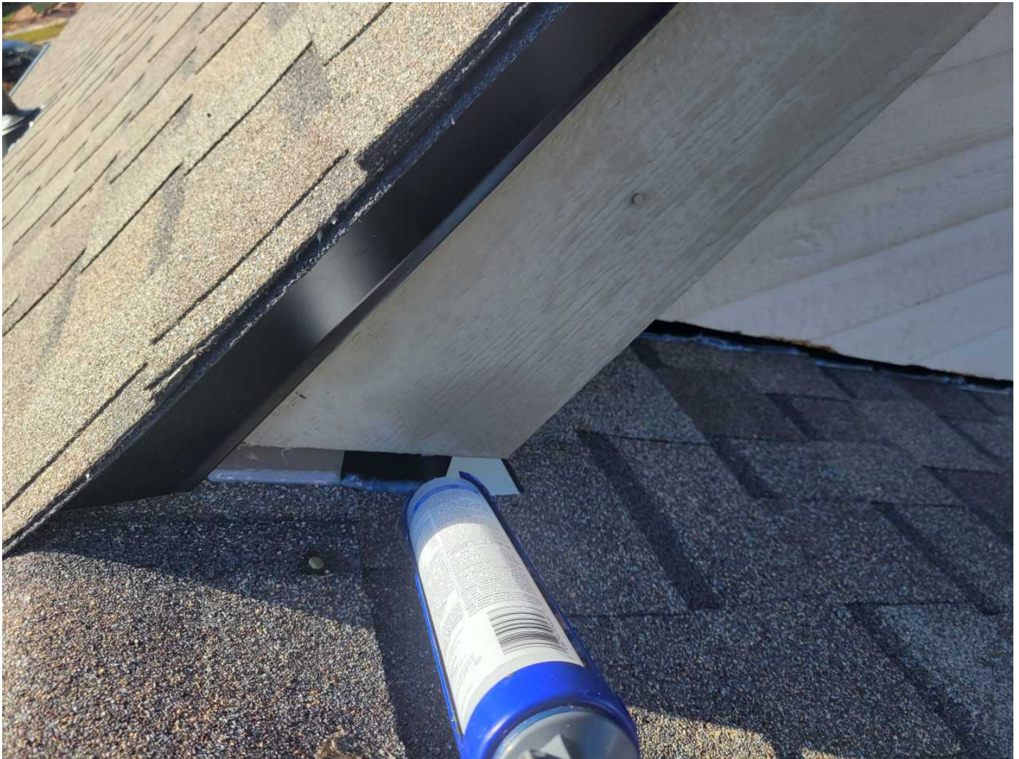
6 7-caulking as existed
