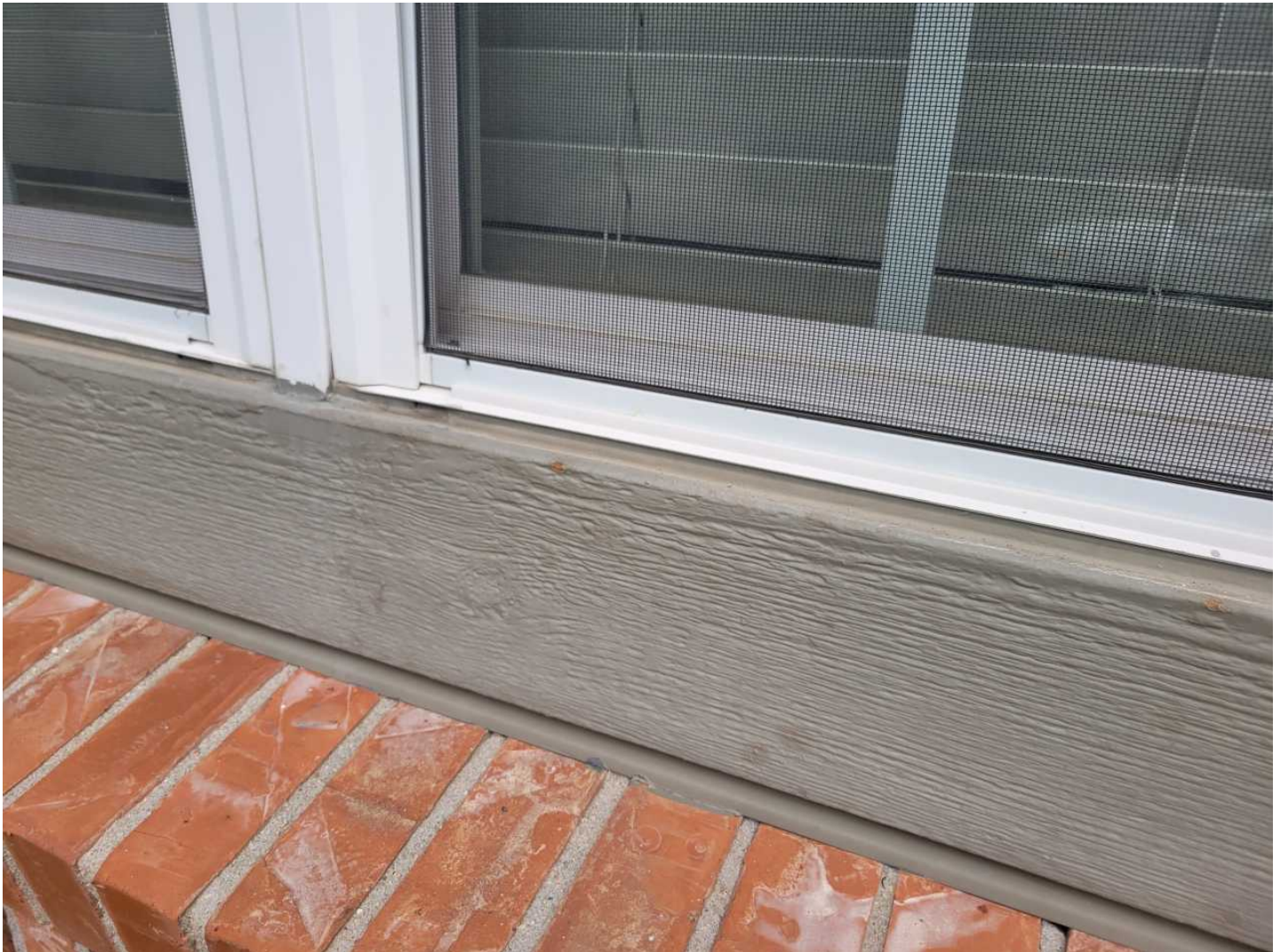
16 17-paint trim front window
