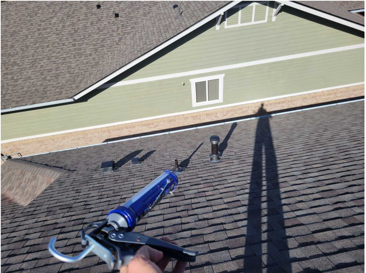
24 25-silicone pipe jacks as existed Date Taken: 10/25/2024
