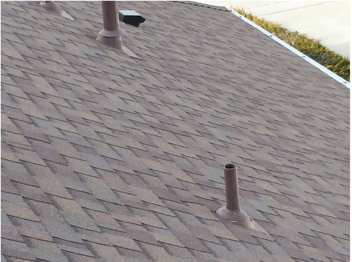
2 3-2014 metal pipe jacks
